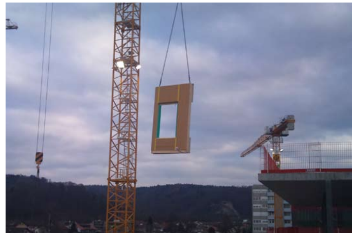
Assembly of elements on building site
